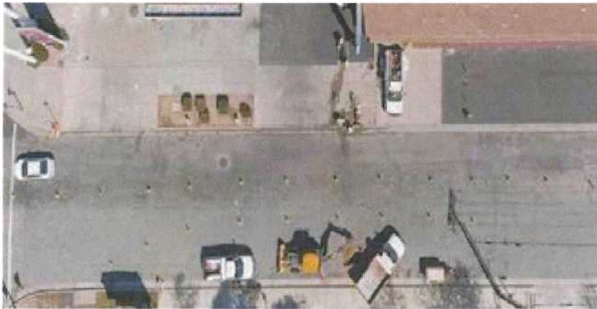
Traffic Control Training - Crews repairing a leak
